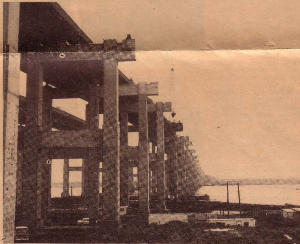
Here is the partially completed span.
